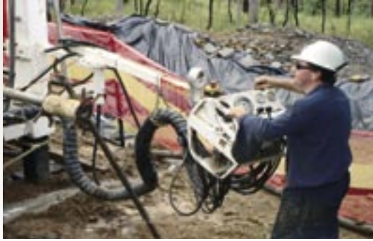
Drilling at Watershed.
