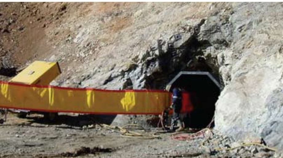
Adit development at Watershed.
