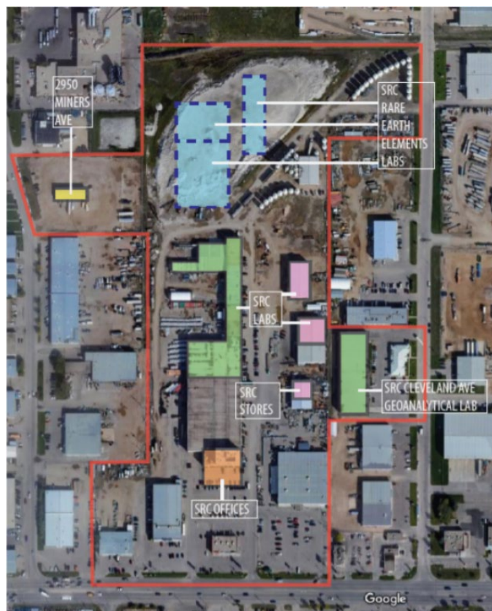
Exhibit 3 – Saskatchewan Research Council’s RE ‘precinct’: VML’s plant is shown adjacent in yellow
