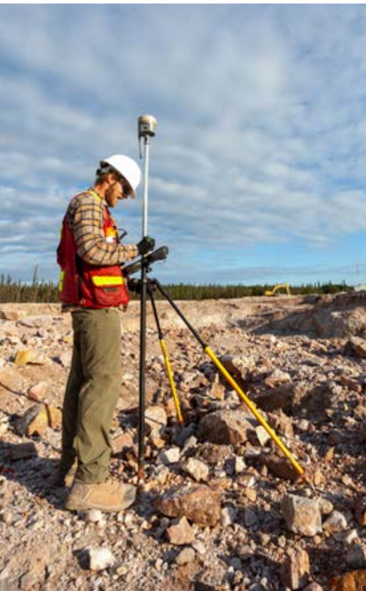
Surveyor Neil Renwick maps a blast pattern at the North T pit face.
